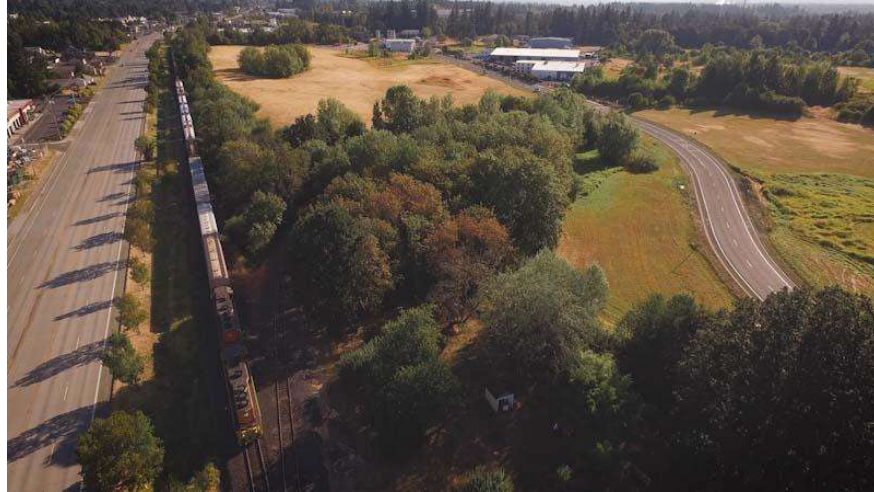
Figure 8. McNulty Creek Industrial Park
