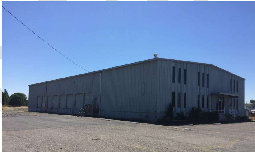
Figure 7. Industrial Building at Milton Creek Industrial Park
